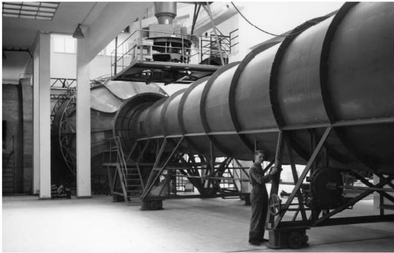
THE HORIZONTAL CLOSED TEST SECTION OF THE SUBSONIC WIND TUNNEL
