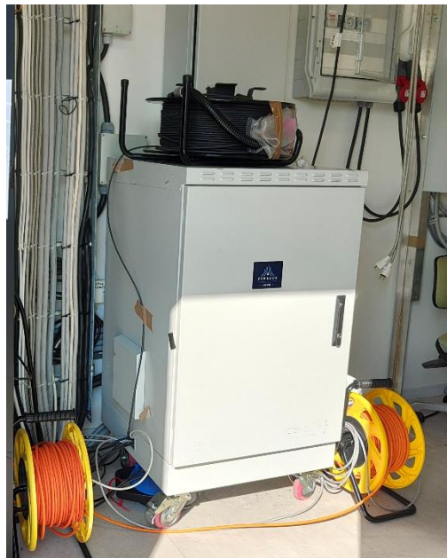
Figure 5 – Electrical support rack of SERA IV placed near of the launch rail inside an electrical container
