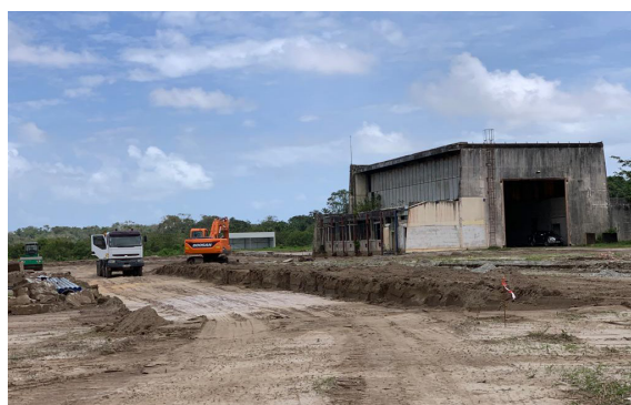
Figure 9 : Civil work around the CALLISTO VPH
