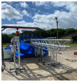
Figure 22: Ramp deployment at Vernon
