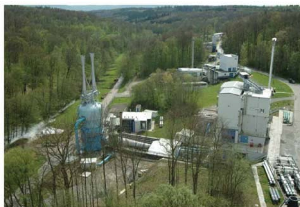
The DLR P4.1 test bench in Lampoldshausen, Germany
