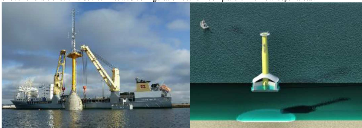
Fig 9 : Ballasted Gravity based foundation
