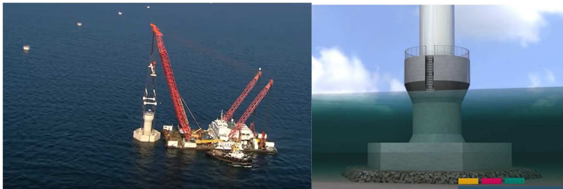
Fig 8 : Gravity based foundation
